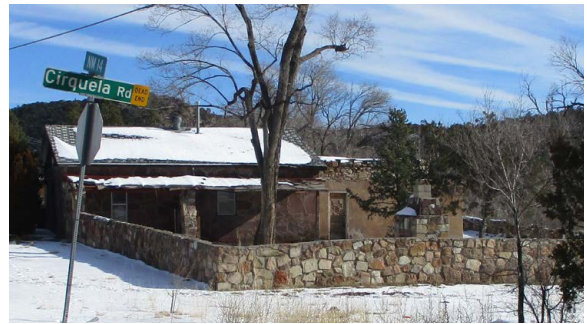
Stone House view from Cirquela Road after grounds clean-up in January. Photo by Rick Holben
